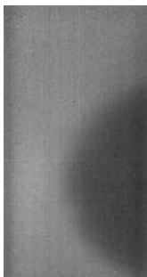
Carbon fiber reinforced polymer (CFRP) delamination.
